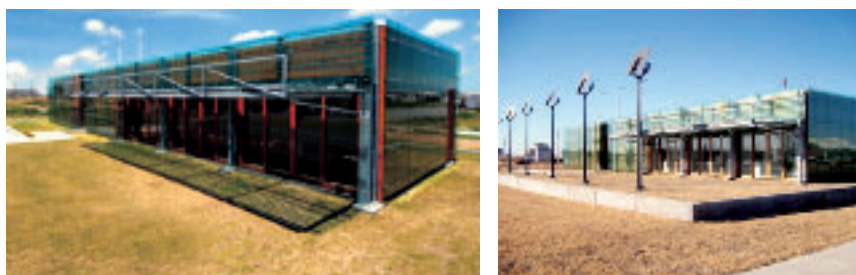
Figure 50 • The 5.4.7 Arts Center, (named after the date of the tornado strike), is the first Leadership in Energy and Environment Design, platinum building in Kansas. It has solar PV panels situated on the ground, eight solar PV panels on the roof and solar lighting installed. The three wind turbines, visible to the rear of the Center, each produce 600 W and are connected to a battery bank
