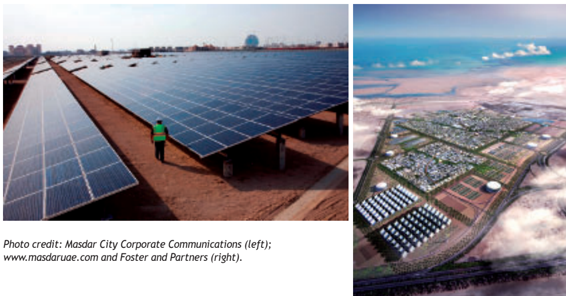
Figure 40 • The 10 MW peak solar PV plant, located on the edge of the planned city (right), is already producing power for use during the first construction phase
