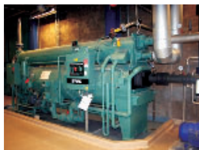
Figure 39 • Woodchips from forest residues are used as the renewable energy fuel in the biomass district heating plant (left). A York adsorption cooling unit in the Väjö Energi AB plant converts heat into chilled water for cooling (right)
