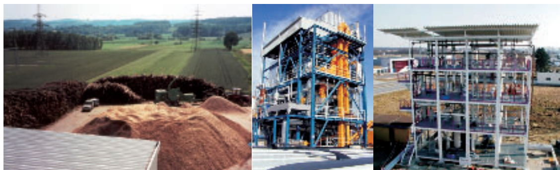
Figure 46 • Biomass resources, collected from the local district (left), are stored at the fluidised-bed, steam gasification, CHP plant (centre). The methanation pilot plant (right) attached to the CHP plant, produces synthetic natural gas and has been operational since October 2008
