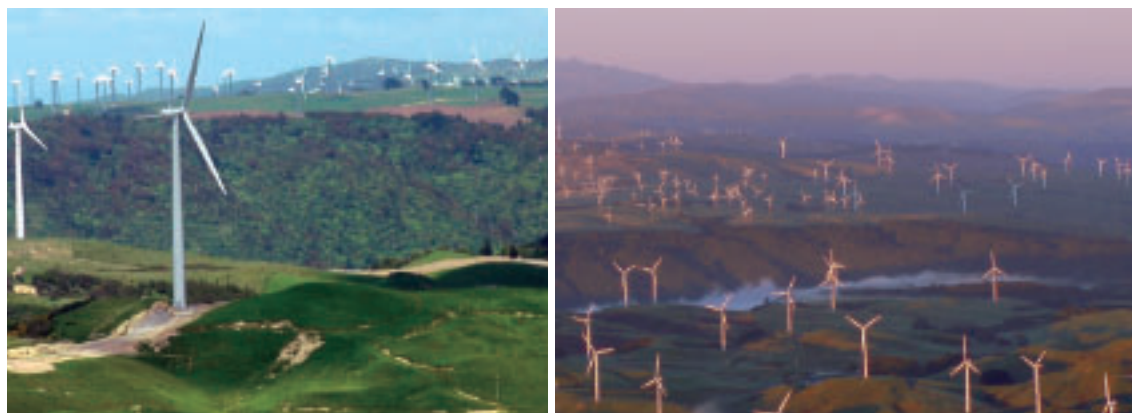
Figure 38 • The 1.5 MW turbines of the 120 MW Te Apiti wind farm under construction (left) and in the foreground (right) are just outside of the Palmerston North city boundary (delineated by the Manawatu Gorge shown by the rising mist). Within the boundary are the original 660 kW turbines of the Tararua wind farm and the 31 recently added 3 MW turbines (seen on the plateau across the gorge). The urban city centre is located 12 km away to the right of the photo, down on the plains
