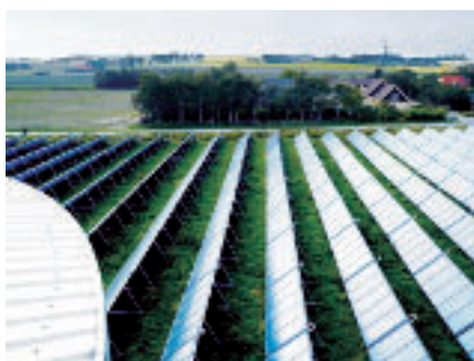
Figure 45 • An array of solar thermal collectors heats water to 70°C, which is then piped to local houses for heating. A wind turbine is visible in the background
