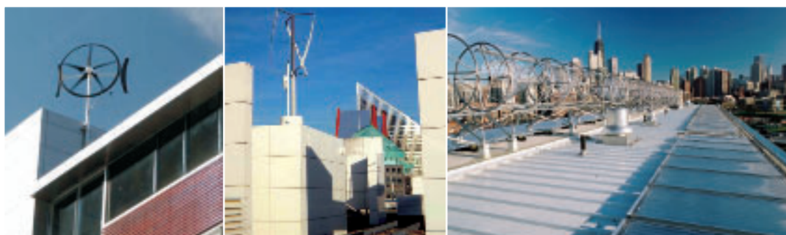
Figure 16 • Examples of roof-mounted micro-turbines include the Swift 2m diameter, horizontal axis, rated at 1.5 kW at 14 m/s wind speed with a ring that reduces noise levels down to 35 decibels (left); the Turby 2.5 kW (at 14 m/s) vertical axis design (centre); and the Aerotecture 1 kW modular system based on a combination of Darrieus and Savonius designs that can be operated horizontally (right) or vertically
