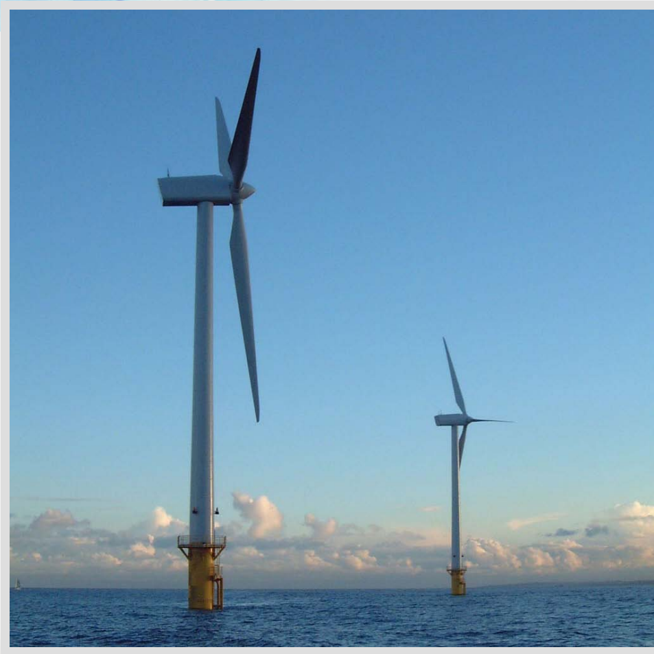
Off-shore Wind turbines, Blyth, U.K.
