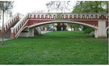
During the construction new materials were used. The concrete strengthened by iron was the invention of Robert Wünsch. The tunnel walls, the slab and a small bridge are built of ferroconcrete. The concrete was mixed by electrical mixers.
