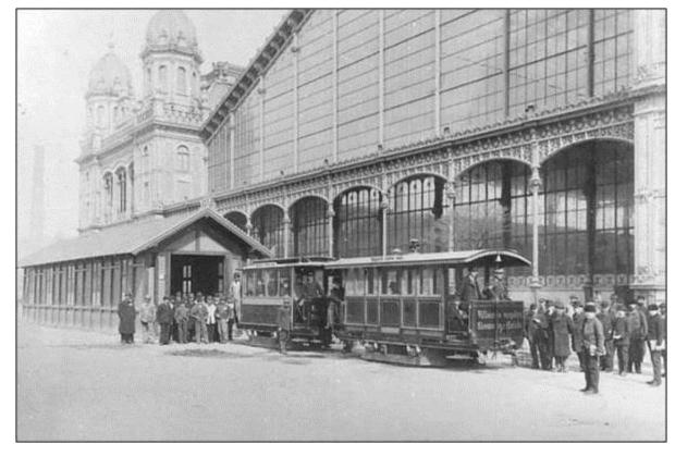
In 1887 a 1000 m track was built by Siemens & Halske for electric tram with lower current collector (sunken below the surface).
