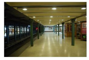
The ferroconcrete ceiling is supported by riveted iron pillars. In 1995 the stations were renovated, fixed, insulated and dyed by anticorrosive painting.
