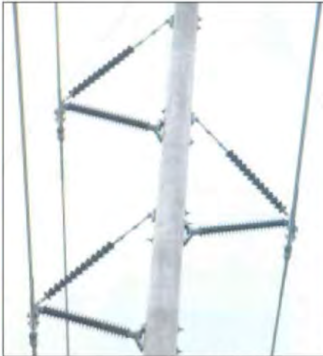
230 kV Compact Lines (USA)
