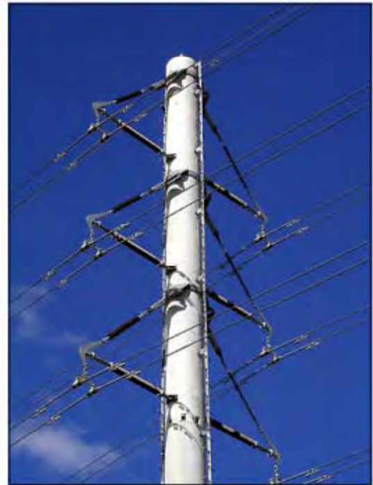
230 kV Compact Lines (USA)
