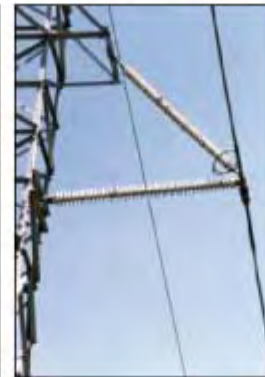
230 kV Compact Lines (USA)
