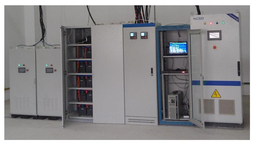
Battery energy storage system, power electronics and control.
